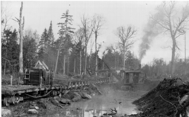
Steam Shovel building railway in the 1920's.
